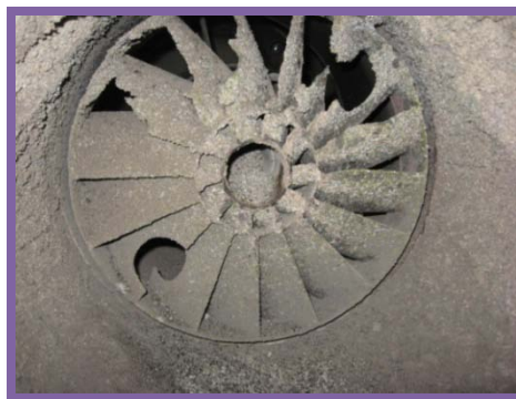
Left: Gas burner diffuser before repairs
