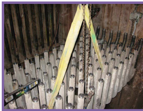
Inconel-protected superheater tubes and headers being lowered to installation location.
