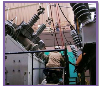
Right: Overhauling a 34,500-volt electrical switch gear
