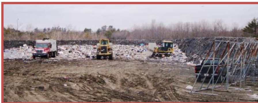
The temporary trash-storage bunker
