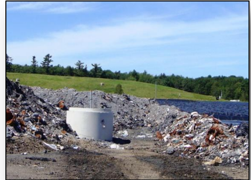
...and, then, the remainder of the pit is filled-in.
