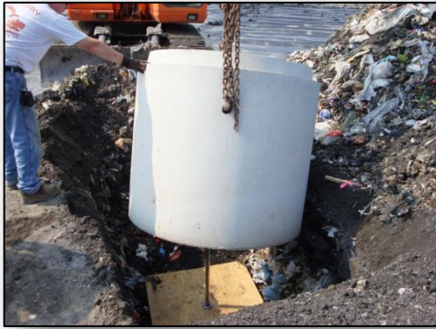
In the next step, a large concrete protective cylinder is placed around the measurement device...
