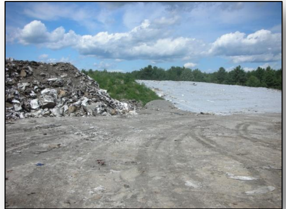
On the left is a pile of wetlap; on the right is the existing MSW storage berm covered with shredded wetlap.
