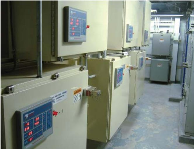
*New electrostatic precipitator controls from Neundorfer contributed to the greatly improved collection efficiency at ecomaine.*
