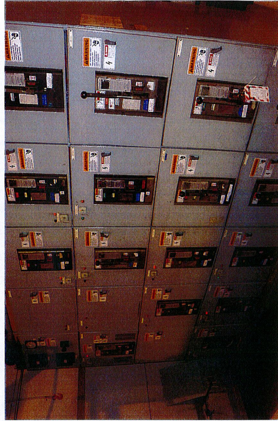
The bottom left photo is of the new low voltage switchgear panel installed during the annual shutdown. The installation was completed within 24 hours. The bottom left photo is of the existing or replaced switchgear panel.
