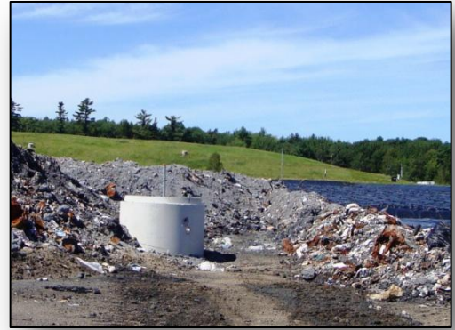
...and, then, the remainder of the pit is filled-in.
