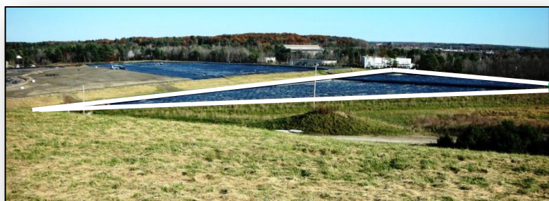
The seven-acre expansion cell (outlined in white) was constructed
