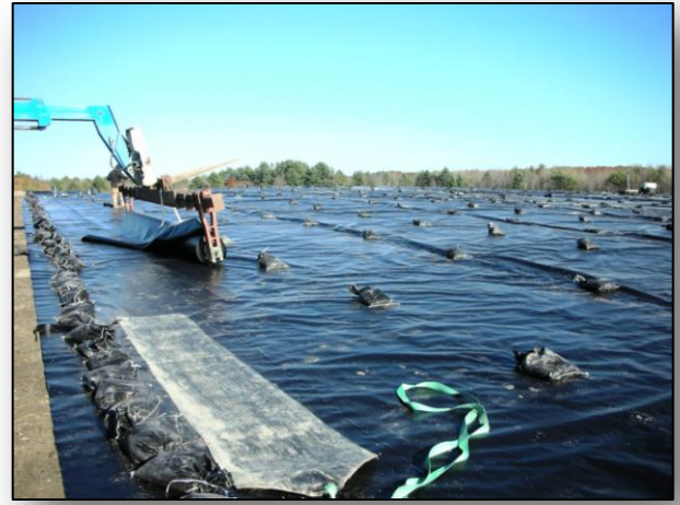
A heavy thick plastic rain cap was placed over the expansion area to keep out the rain. You can see a sample of this material on display at the tent.
